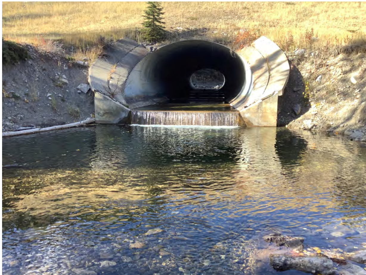
Photo 7.5 Looking upstream at outlet of existing culvert under Highway 66
