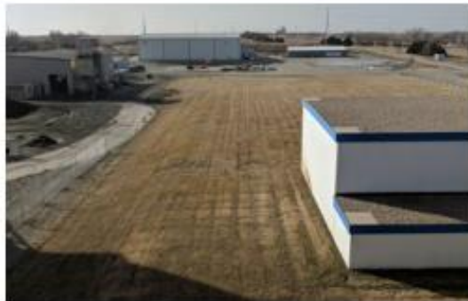
Capped mound of Hallam facility
