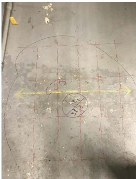
Location of Core C23 after GPR scanning
