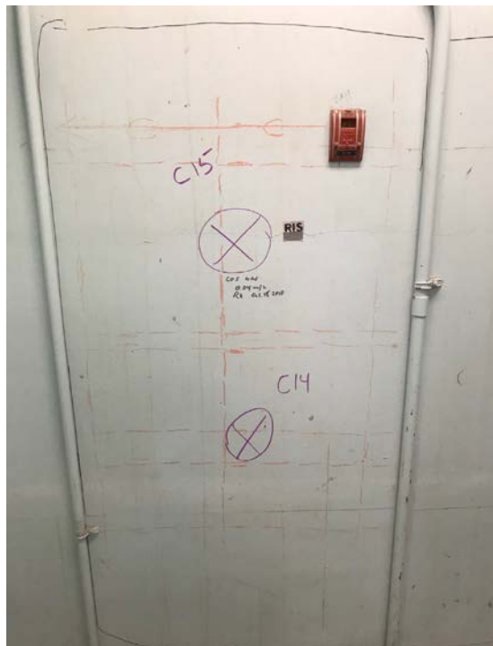
Location of Cores C14 and 15 after GPR scanning
