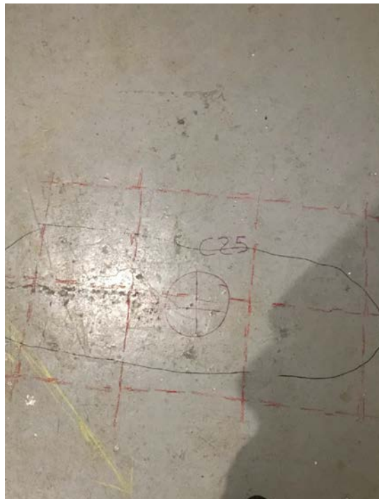
Location of Core C25 after GPR scanning
