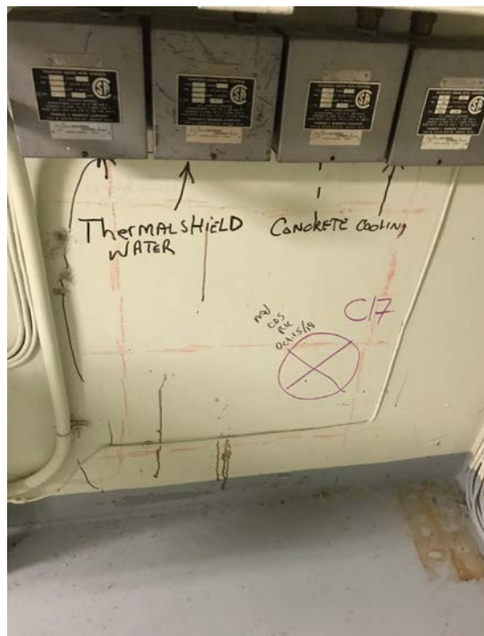
Location of Core C17 after GPR scanning
