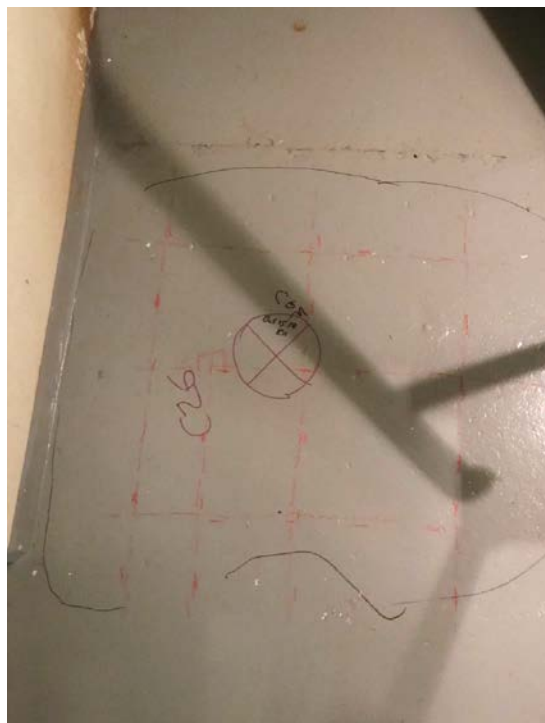
Location of Core C26 after GPR scanning
