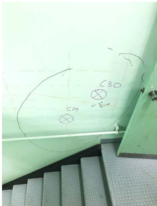
Location of Cores C29 and 30 after GPR scanning
