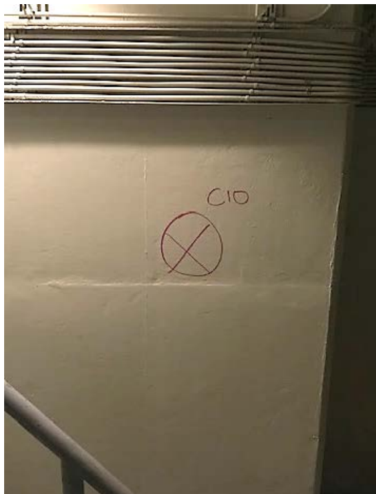
Location of Core C10 before GPR scanning
