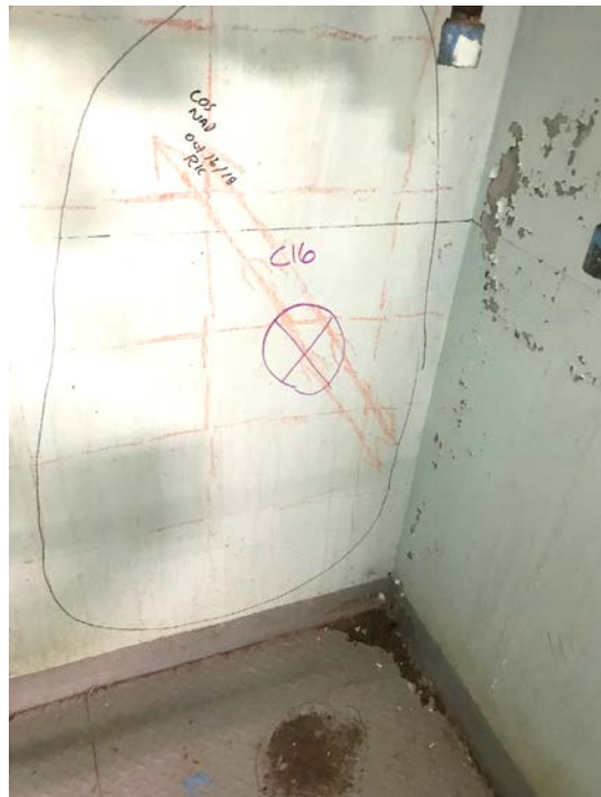
Location of Core C16 after GPR scanning
