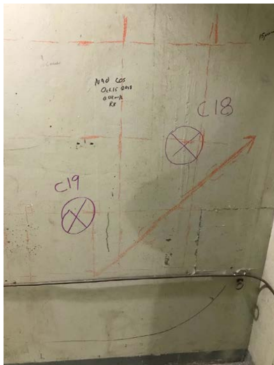
Location of Cores C18 and 19 after GPR scanning
