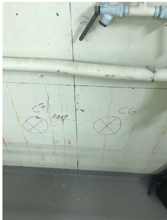
Location of Cores C6 and C7 after GPR scanning
