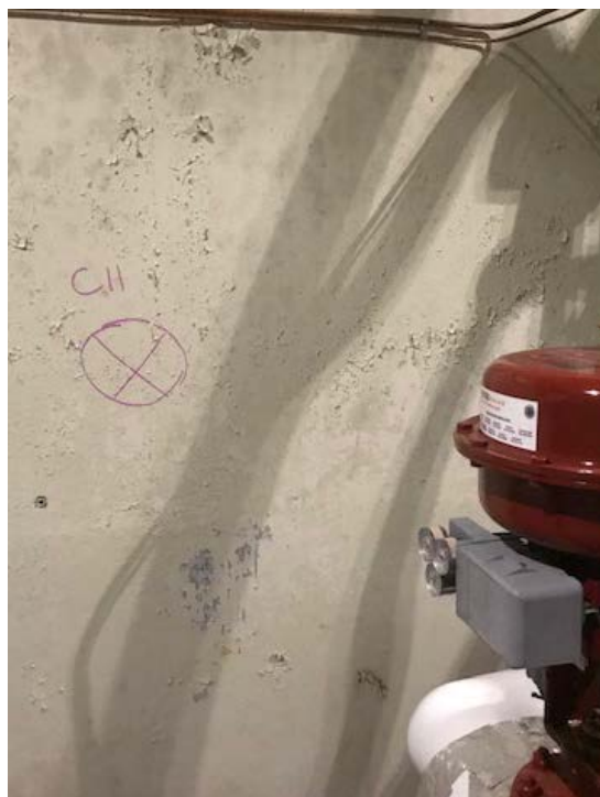
Location of Core C11 before GPR scanning
