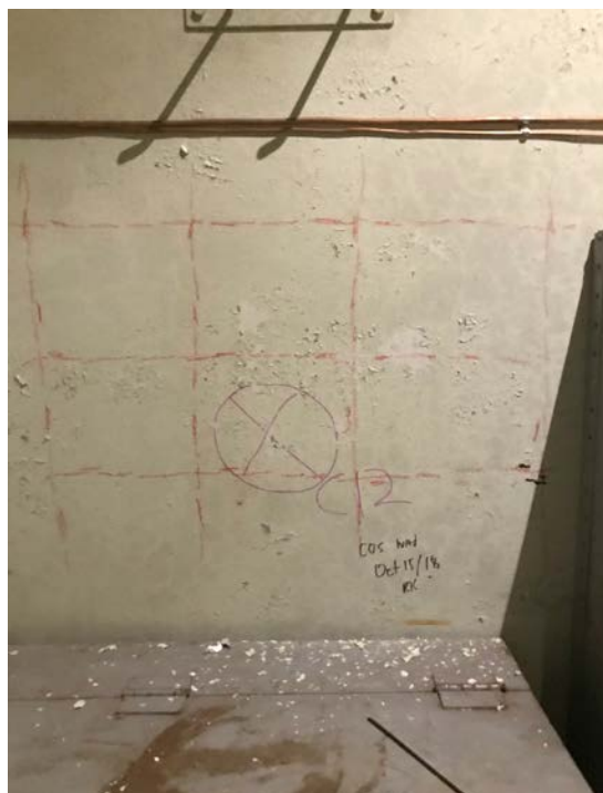
Location of Core C12 after GPR scanning
