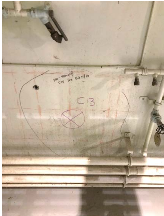
Location of Core C13 after GPR scanning
