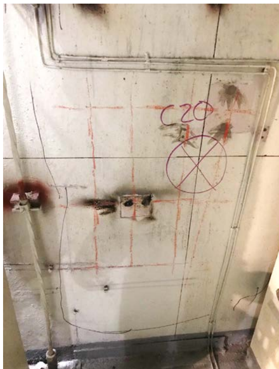
Location of Core C20 after GPR scanning
