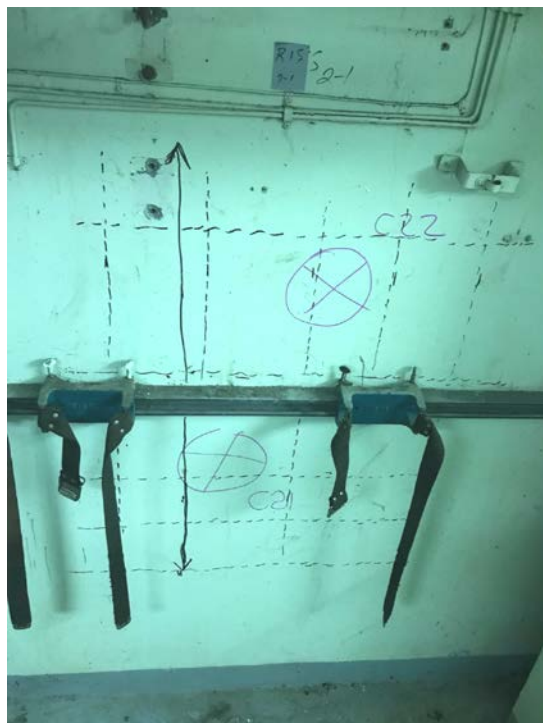
Location of Cores C21 and C22 after GPR scanning
