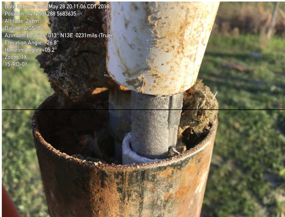
Figure 5: 15-RD-01, showing broken standpipe; obstruction also present at 1.497 m.
