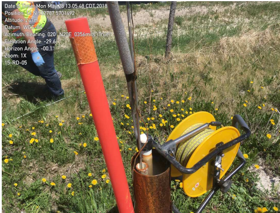
Figure 3: 15-RD-05, showing damaged lower standpipe. The foam insert could not be removed further due to damage to standpipe below.
