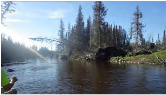
22+000: Erosion and fallen trees on the right bank approximately 230 m downstream from 22+000 (2014).
