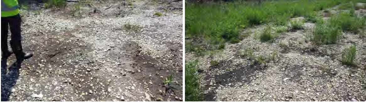
14+500: Bare area on right side of creek in 2013 (left) and 2014 (right).
