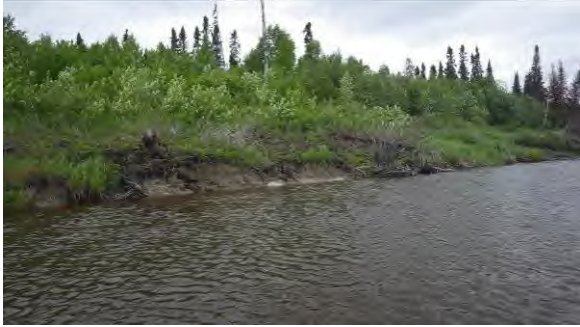
26+500: Erosion on right side of creek approximately 175 m downstream from transect (2014).
