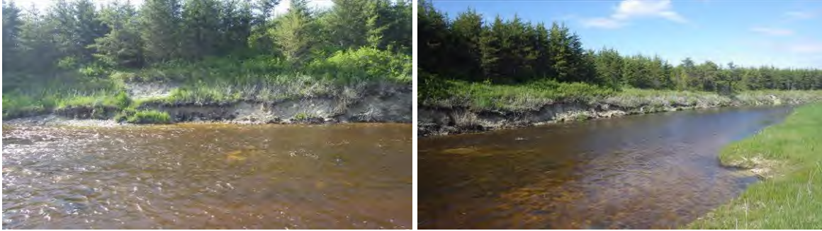
16+000: Erosion on left side approximately 50 m downstream from 16+000 (2014).
