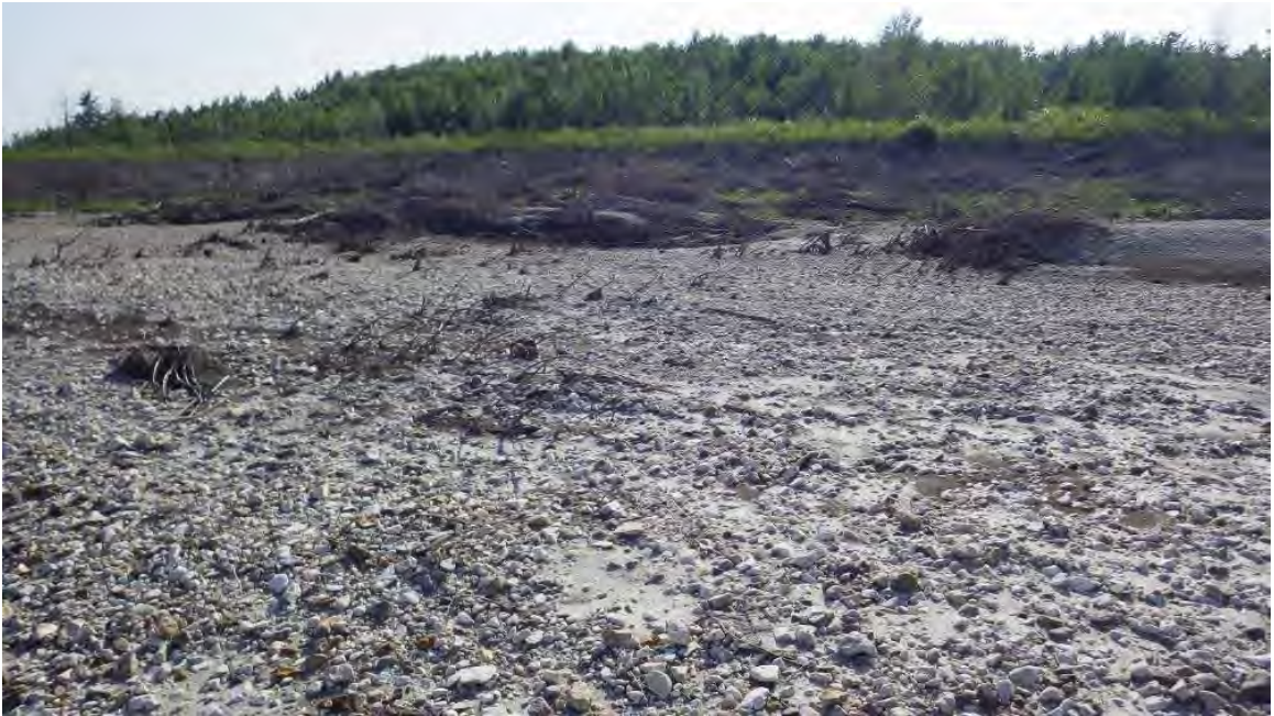
Photo 1. "Bare" substrate observed at 18+000.
