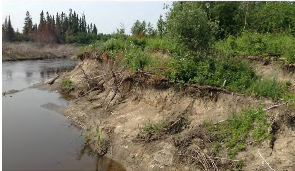
Photo 13. Slump on left side of creek at 25+000 (looking upstream).
