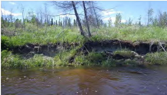
19+000: Erosion on left side of creek approximately 100 m upstream (2014).
