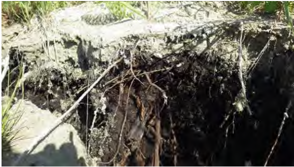
16+500: Right bank: Deposition above eroding bank.
