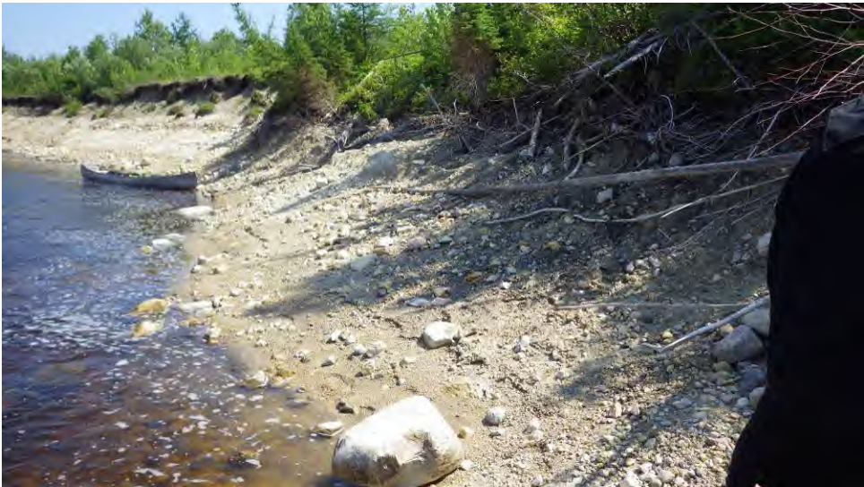
Photo 7. Steep bank along Buffalo Creek at 15+000.
