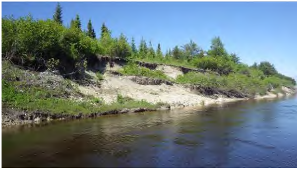
15+000: Erosion on left bank approximately 360 m downstream from 15+000 (2014).
