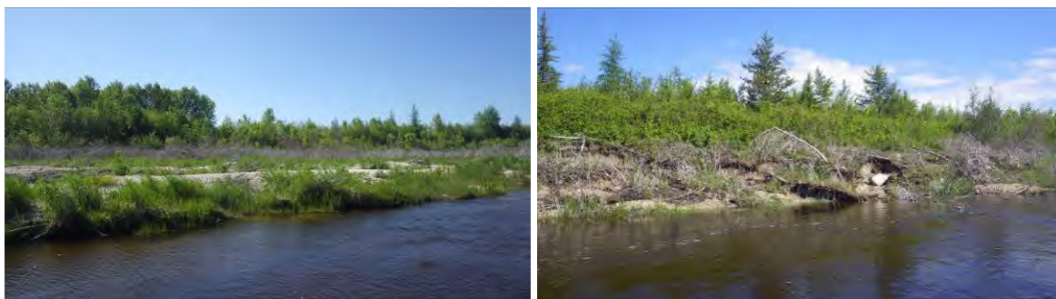
16+000: Deposition on left side (left) and erosion on right side (right) approximately 150 m upstream from 16+000.
