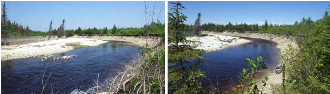
15+000: On right side of creek, looking downstream in 2013 (left) and 2014 (right).
