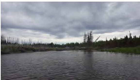
25+500: Area of erosion on left side of creek approximately 175 m upstream from transect (2014).
