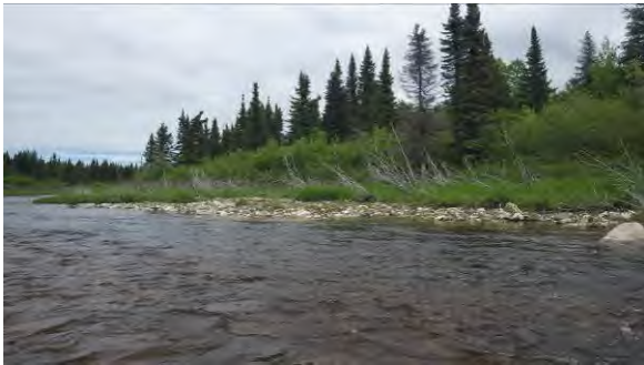
14+500: Erosion on right side approximately 175 m upstream from 14+500 (2014).
