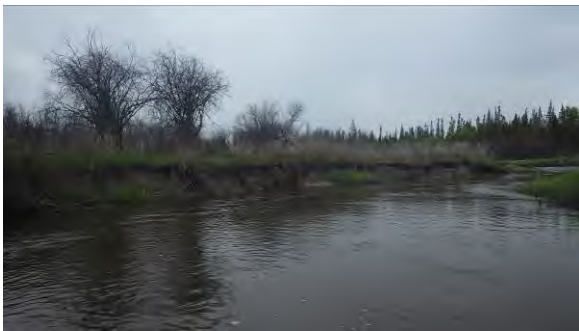
26+000: Area of erosion on left bank approximately 250 m upstream from transect.
