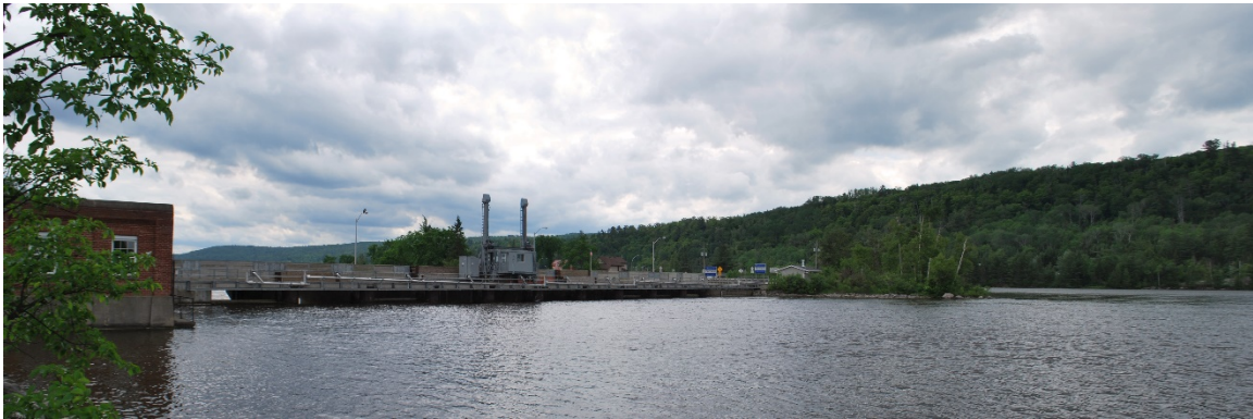
Photo 2 : Timiskaming Dam-Bridge of Quebec – view from upstream
