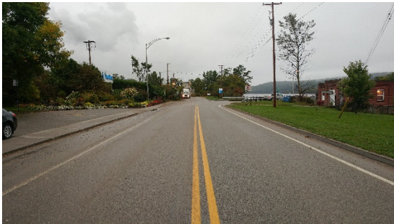
Photo 9 : Dam entrance, Kipawa Road - view toward the south
