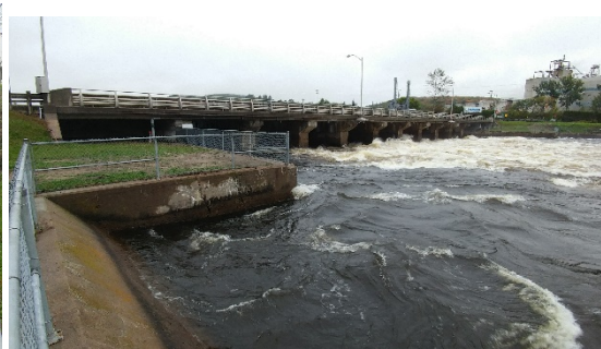
Photo 6 : Right bank – view from downstream
