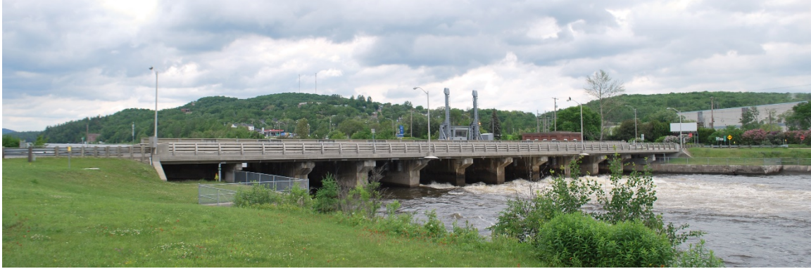
Photo 1 : Timiskaming Dam-Bridge of Quebec – view from downstream
