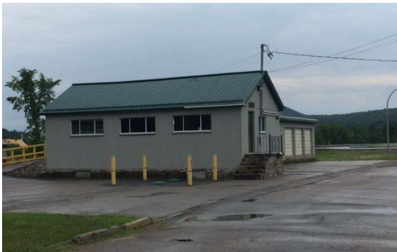
Photo 13 : PSC garage, Long Sault Island
