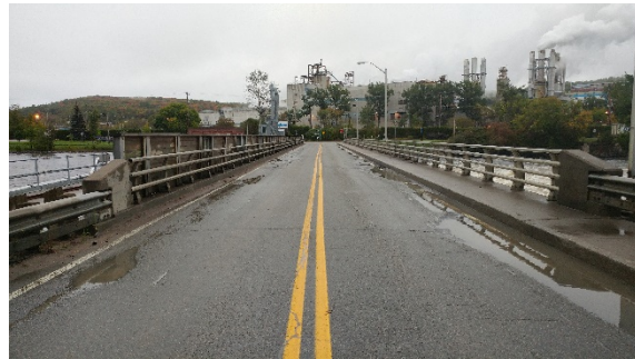
Photo 10 : Dam deck, roads 63 et 101 - view toward the east
