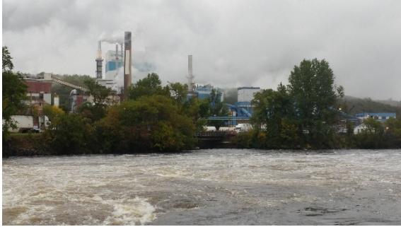
Photo 7 : Left bank downstream - Mouth of Gordon Creek
