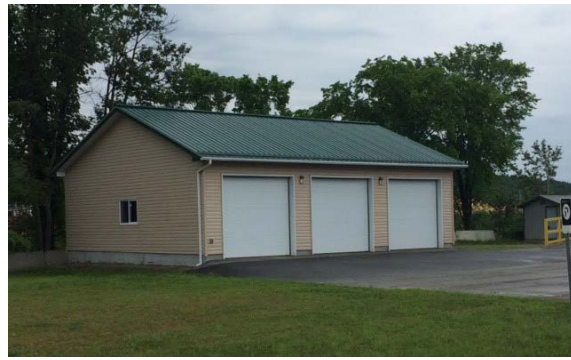
Photo 14 : Garage, Long Sault Island
