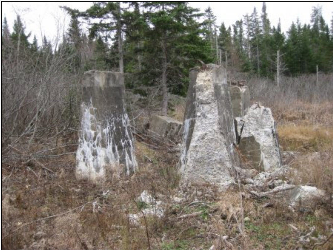
Concrete foundation to the south of the gravel access road
