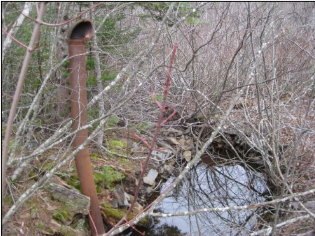
Typical water filled excavation, potential shaft
