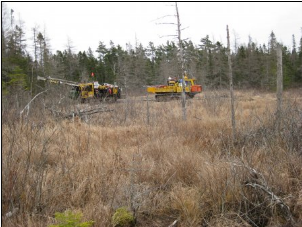
Typical drill operation setup in the area of the proposed pit
