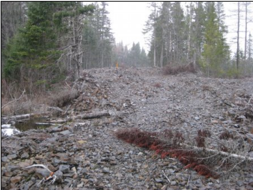
Graded waste rock along the western edge of the proposed pit
