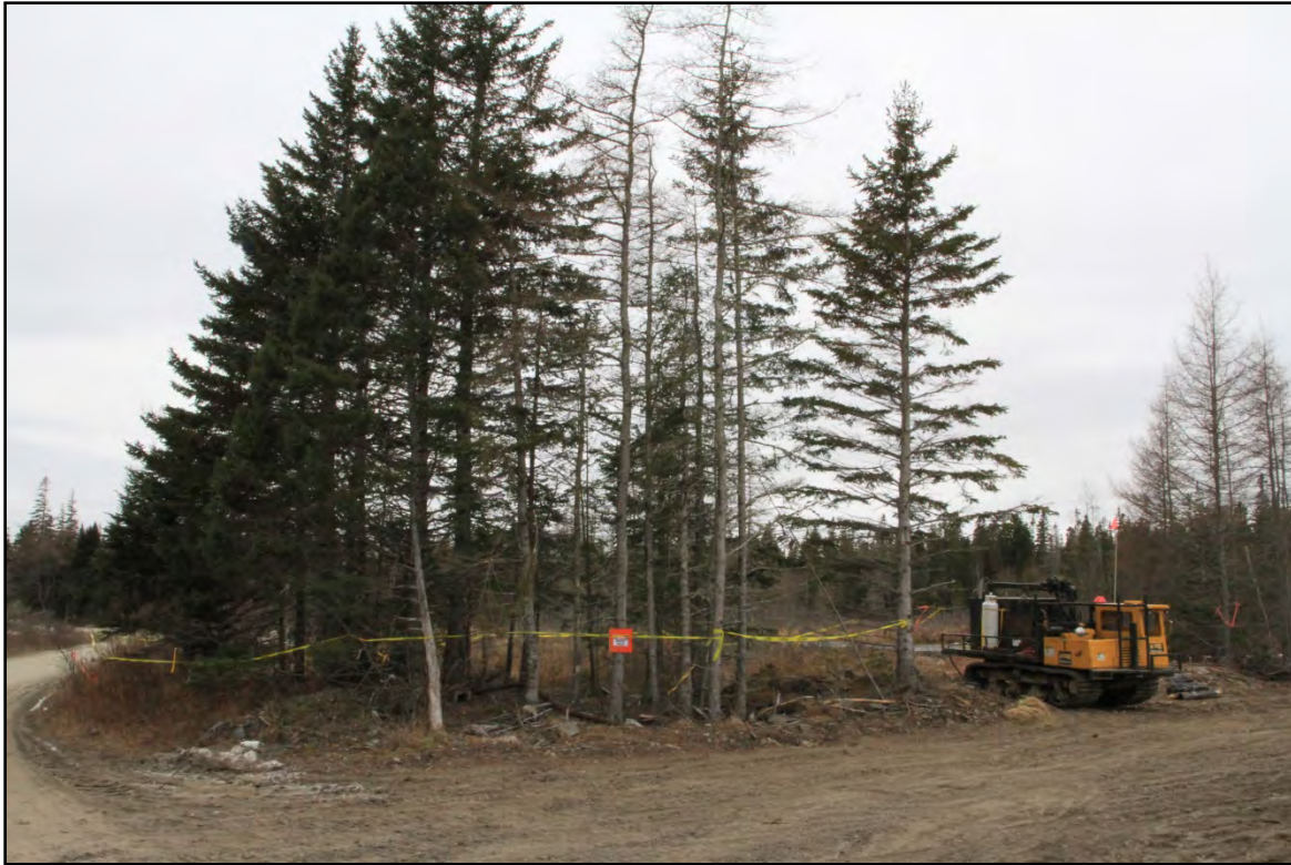
PLATE 23: Site 5 as seen during 2018 reconnaissance. Facing northwest; December 8, 2018.
