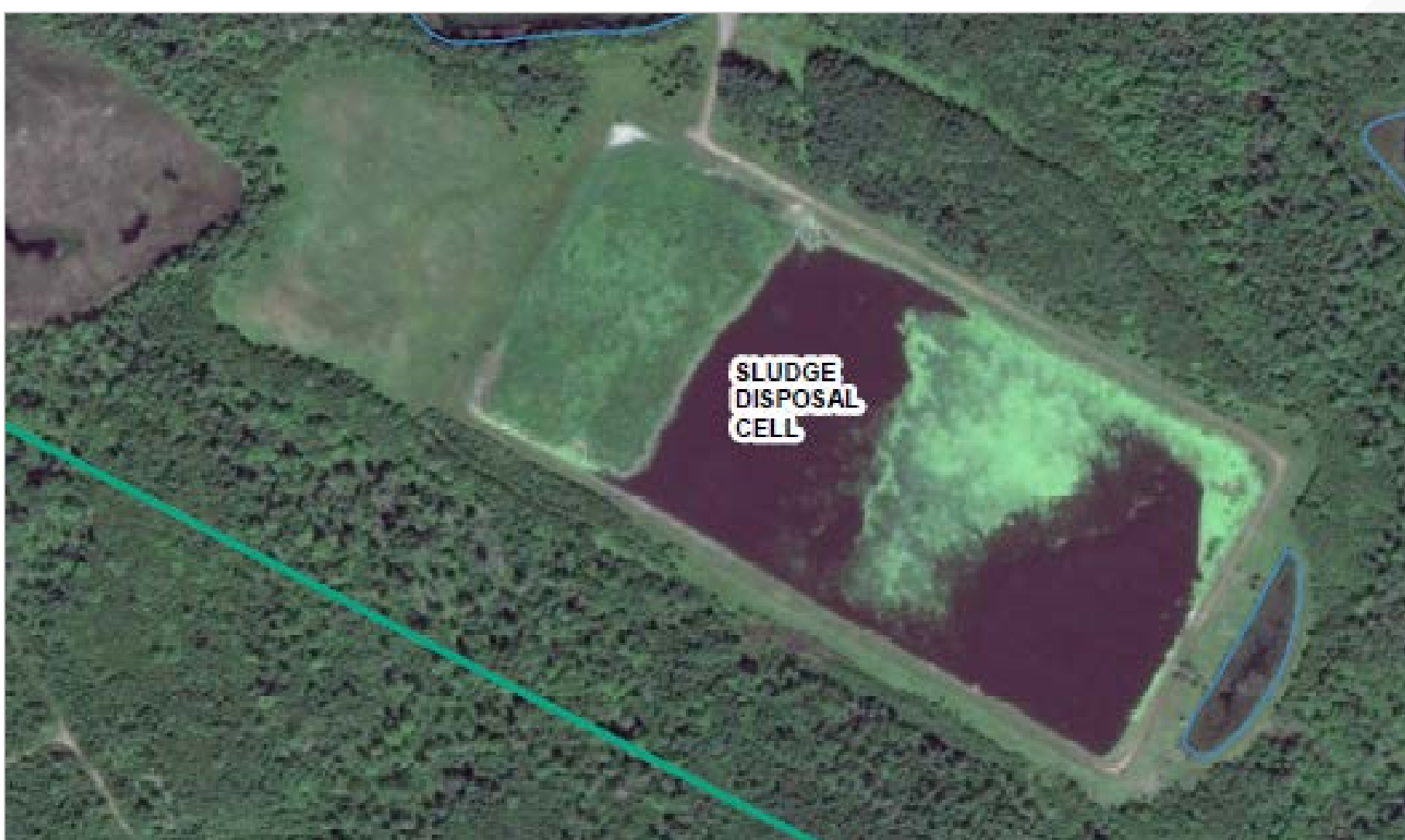
Existing Sludge Disposal Cell
