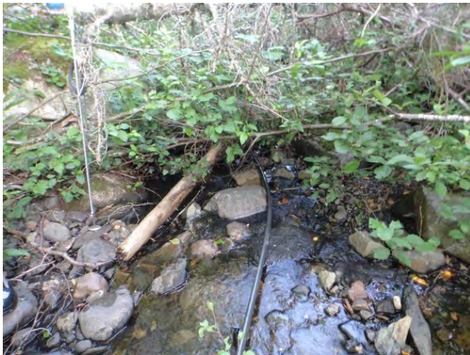
Photo 103 Stream Crossing C001a 0 to 50 m Upstream Facing Downstream
