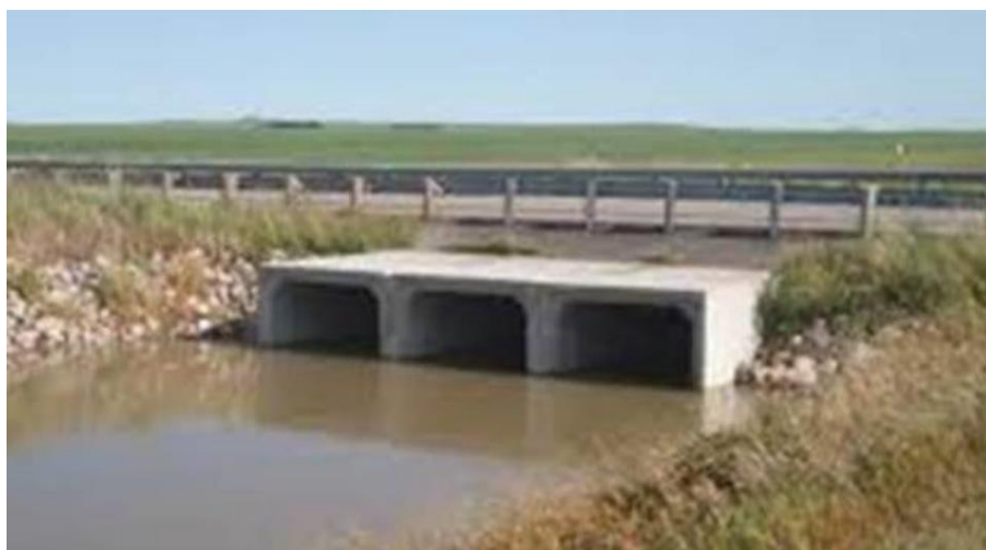
Figure 2-38 Type 3 - Box Culvert
