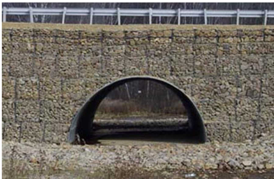
Figure 2-37 Type 2 - Arch Culvert
