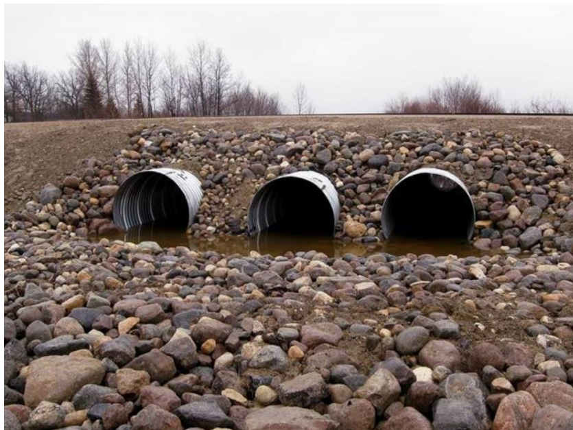
Figure 2-39 Type 4 - Round Pipe Culvert
