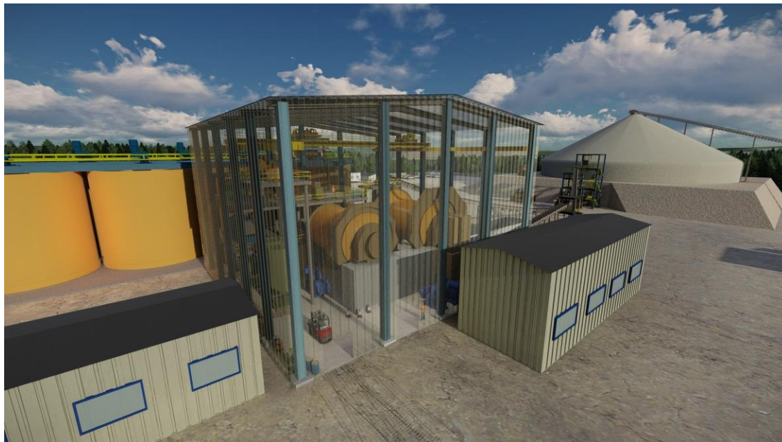
Figure 2-26 External View of the Grinding Mill Building (exterior cladding shown as transparent for illustrative purposes), adjacent to the Leaching Tanks, Reagents Preparation Building and Gold Room, with Stockpile in the distance
