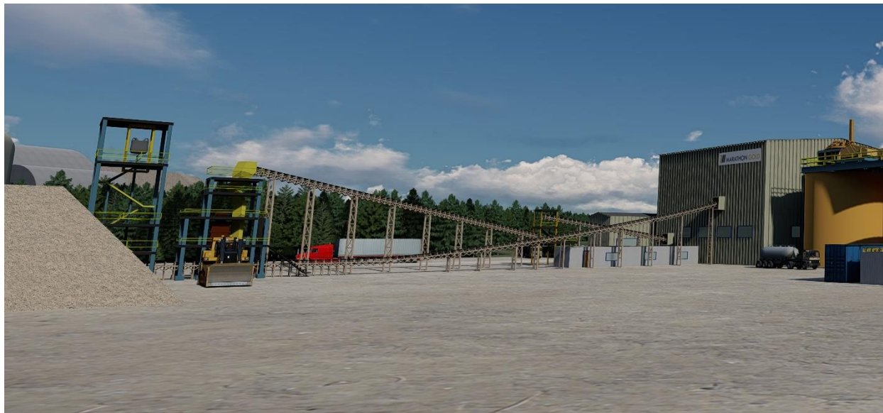
Figure 2-21 Crushing Area (conveyors illustrated without planned enclosures)
