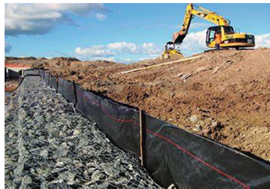
↑ Reducing Project Effects (Mitigation) with the Silt Fence
