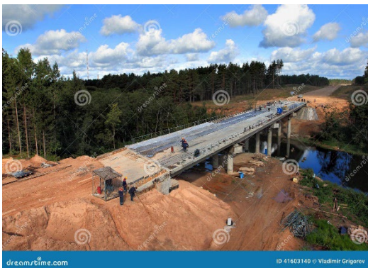
↑ Project Effects: Corrosion (soil loss)
