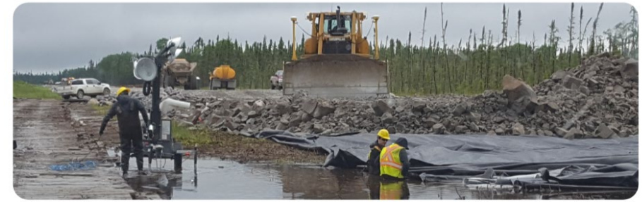
Construction photos courtesy of Dillon Consulting, AECOM and KGS
