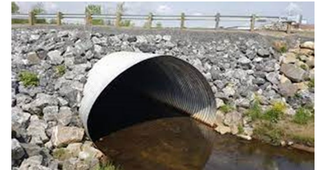
Steel Arch Culvert
