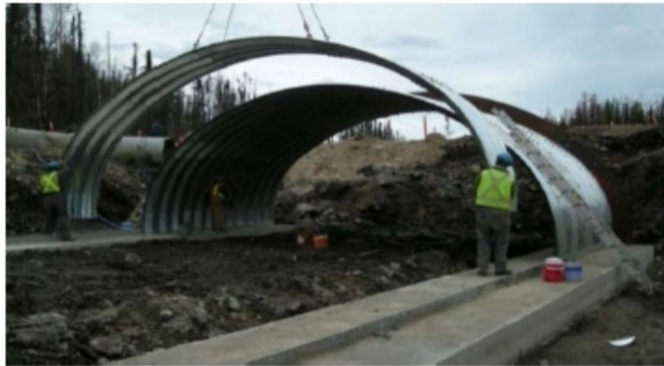
Open Bottom Steel Arch Culvert Under Construction
