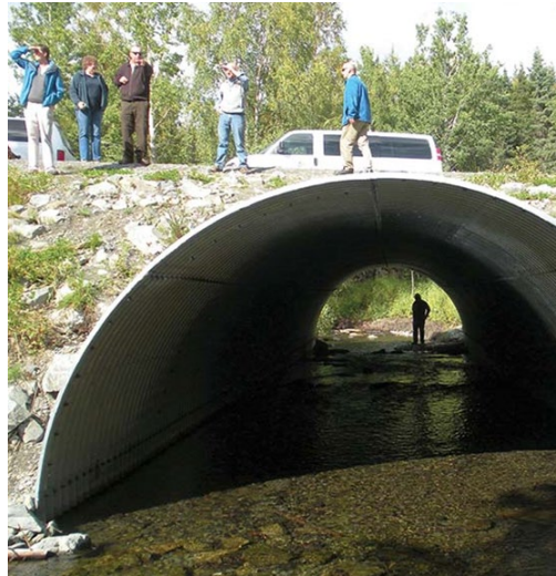
Open Bottom Steel Arch Culvert In Service
