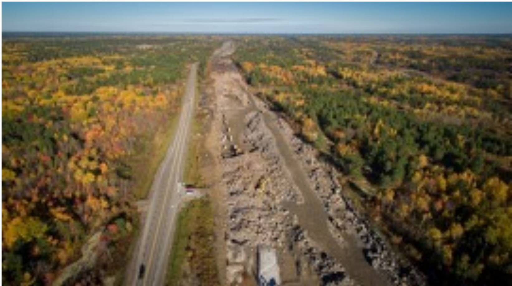
New highway construction near French River, ON.
