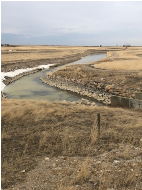
Photo 7 Phase 3 - Inlet Canal from SMRID Main Canal to Horsefly Reservoir
