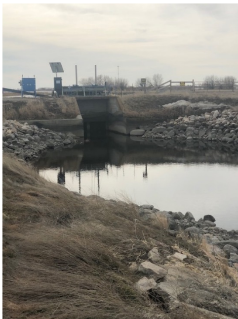
Photo 1 Phase 1- Taber Lake Outlet Structure
