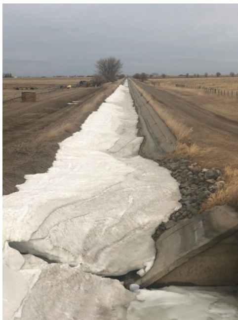
Photo 2 Phase 1 – Beginning of Channel Drain Looking West
