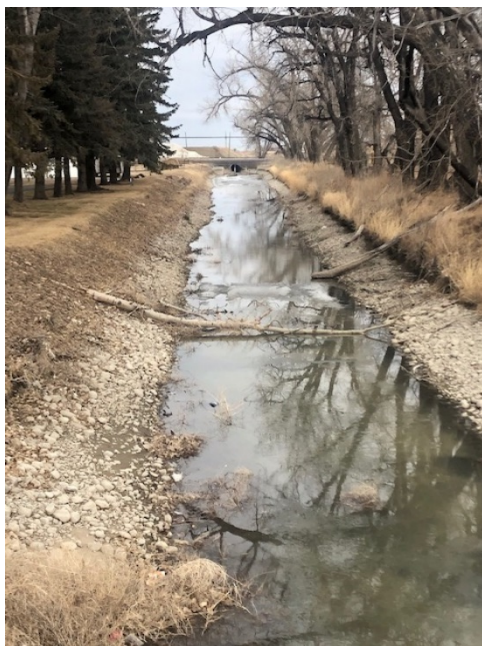
Photo 6 Phase 2 – Horsefly Canal Looking North, Highway 3 Crossing in the Distance
