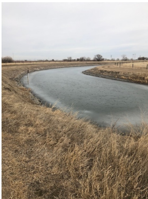
Photo 5 Phase 2 – Horsefly Outlet Channel Looking North
