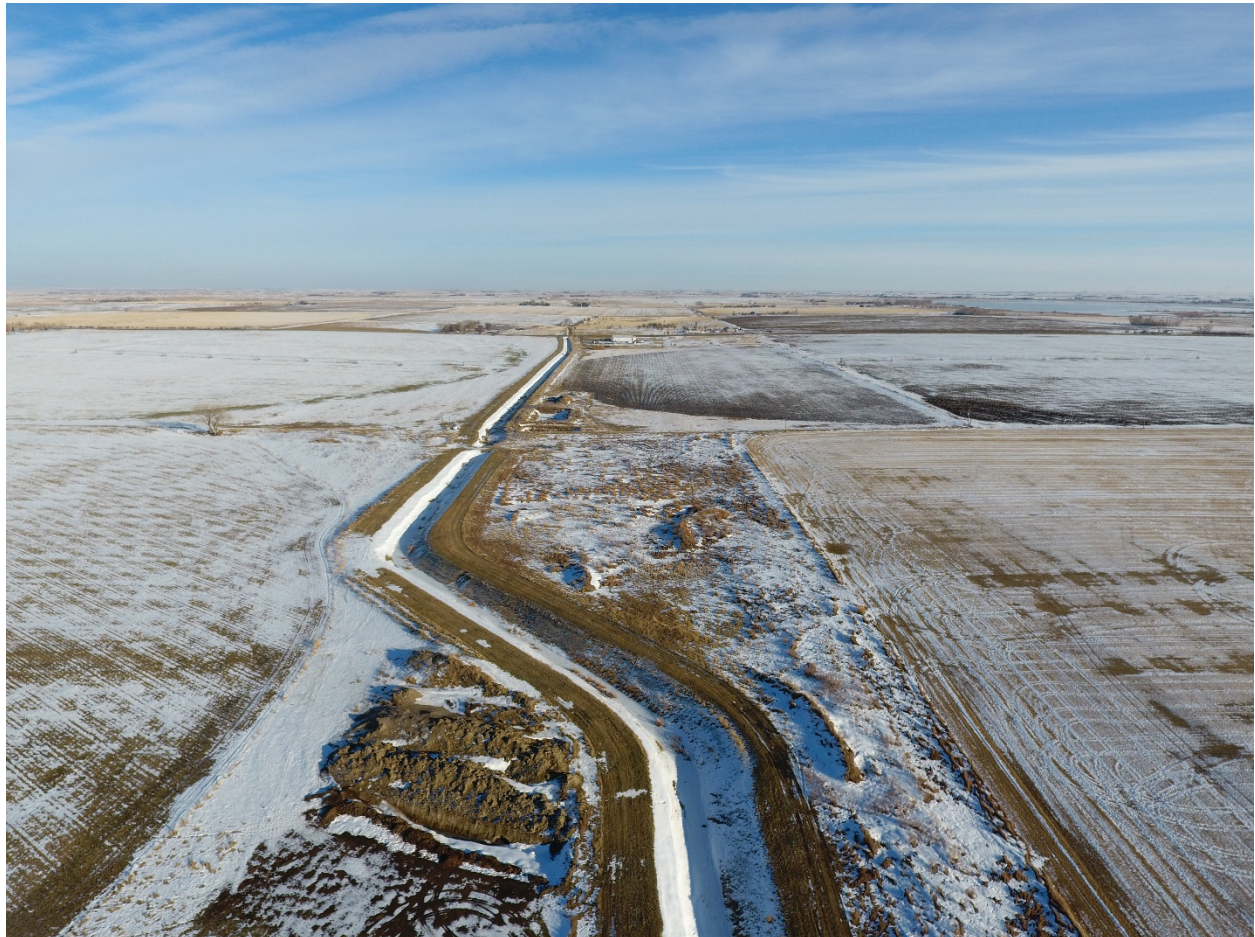
Photo 3 Phase 1- Channel Drain Looking East; Taber Lake in Right Background
