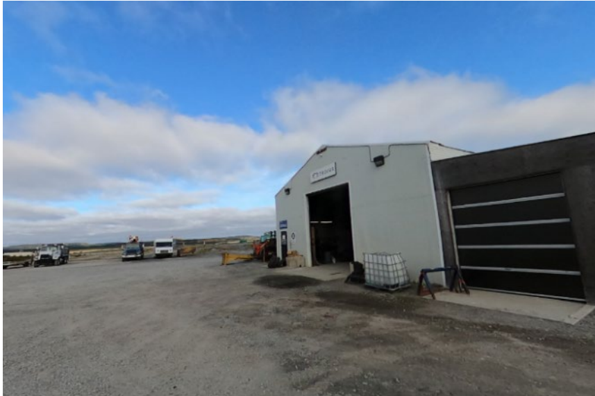
Photo 23.11 Warehouses for Workplaces, Stantec, October 2023
