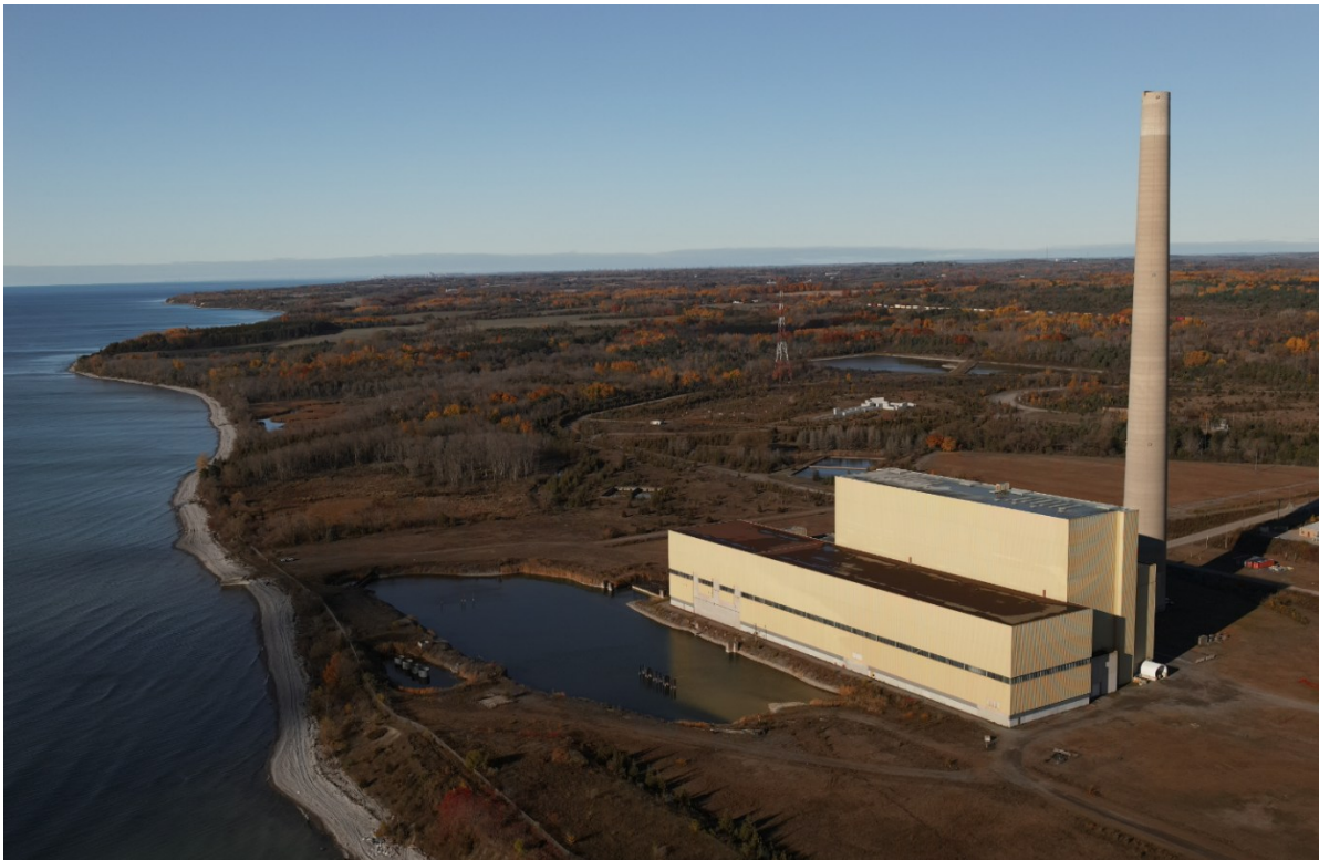
Figure 5: Existing Wesleyville Powerhouse and Chimney Stack
