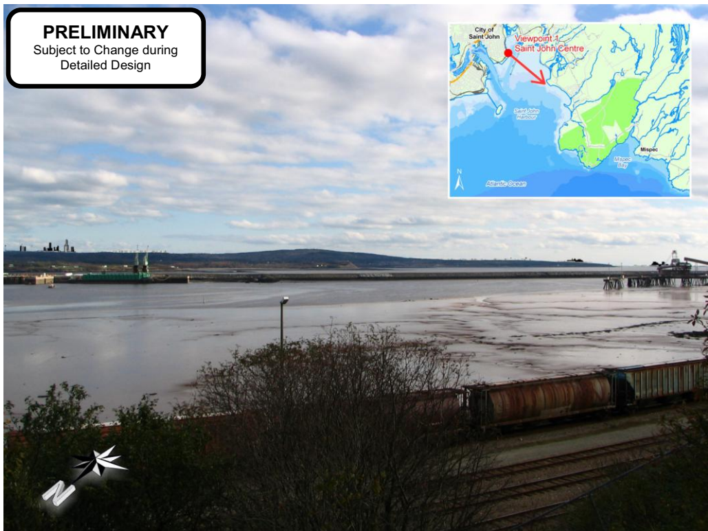
Figure 3.9 3-D Photo Montage of Marine Terminal from Crown Street, Saint John (Viewpoint 1)
