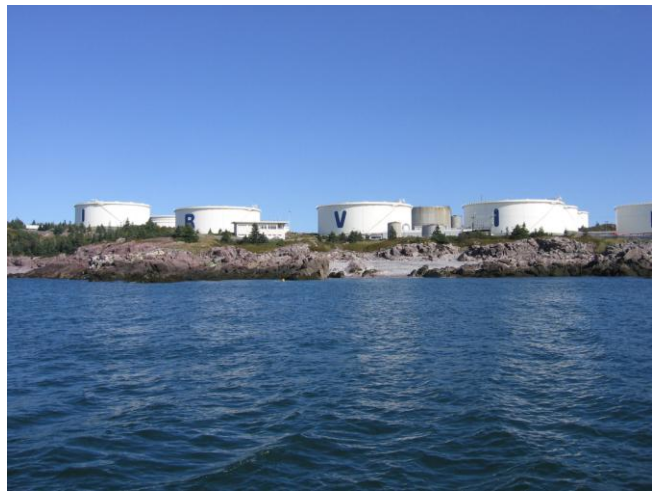
Figure 10.9 Ramped and Irregular Bedrock Shoreline West of Mispec Point at the Canaport Facility
