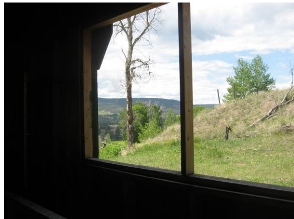
Photo 34. Open window frames
