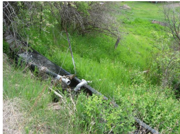
Photo 8. Irrigation pipe in upstream water supply ditch
