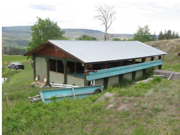
Photo 13. Hatchery NE view
