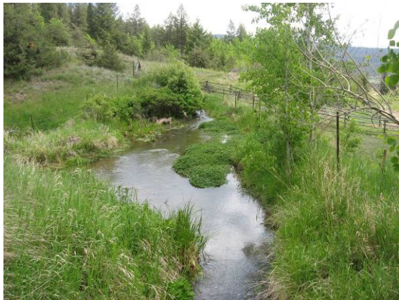
Photo 7. Upstream water supply ditch
