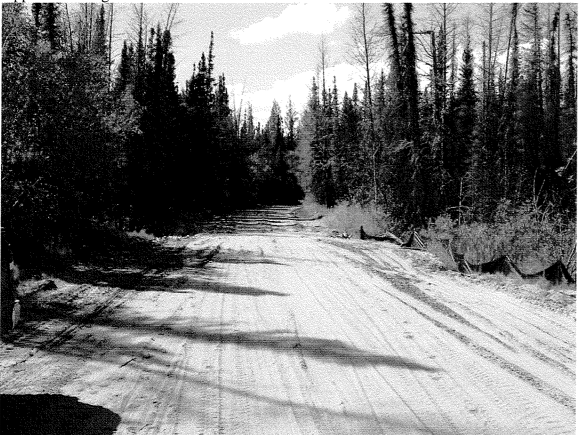
Approach facing west
