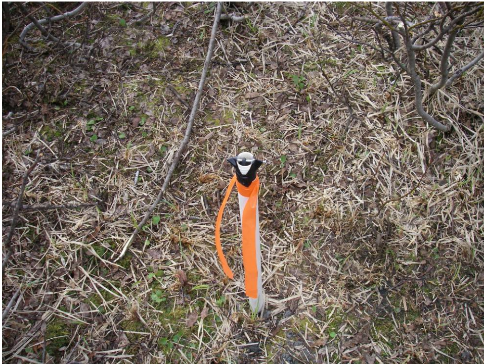
b) Well installation. A hand auger was used to dig holes, and flagging tape was used to facilitate site identification. Where appropriate, water level instrumentation was installed inside the well. Photo taken: June 2008.
