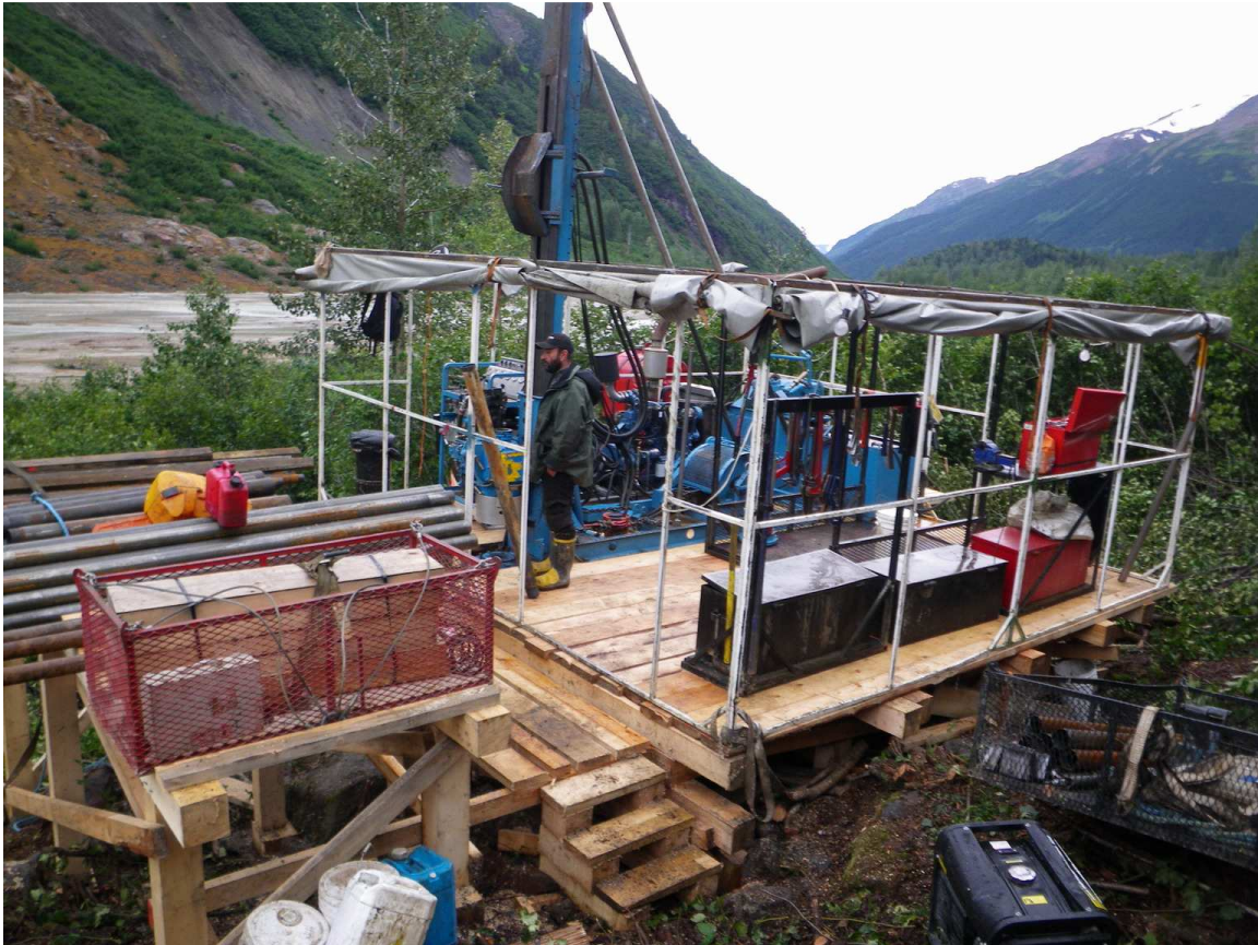
Figure 2.7 Hy-Tech Geotechnical Drill Rig in Mitchell Valley at KC09-09
