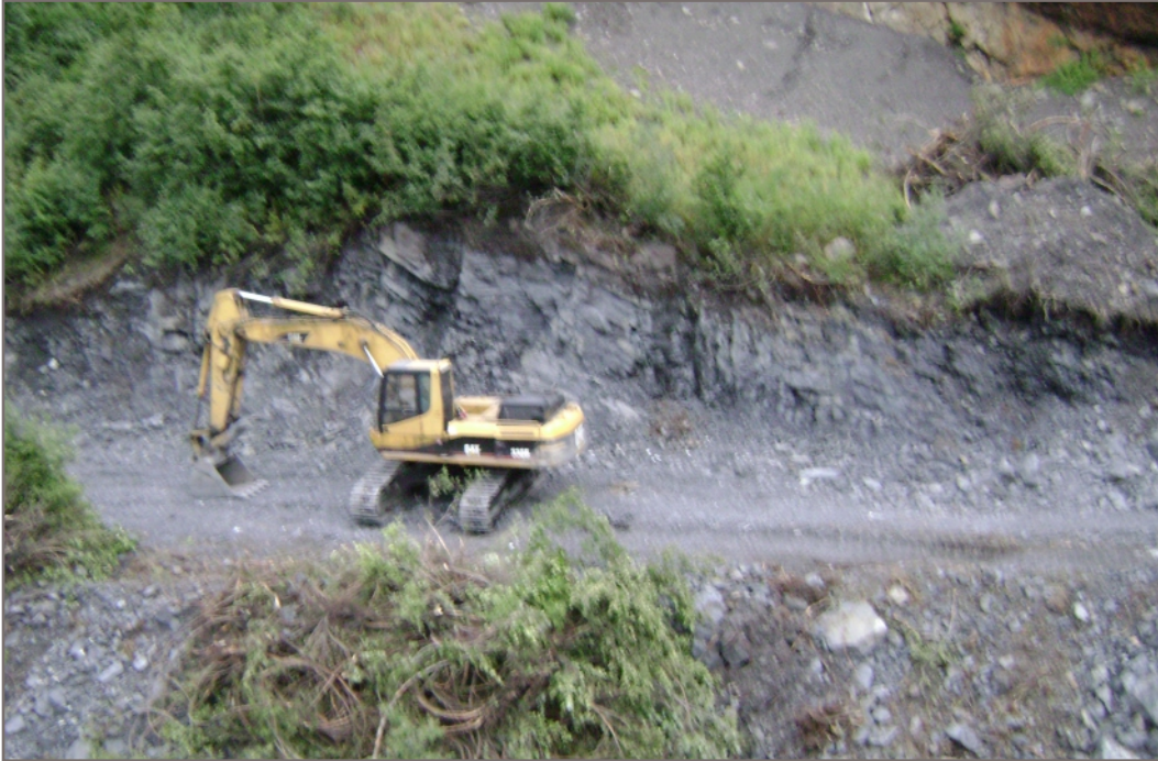
Photo 7: The backhoe on a portion of Pretium's newly constructed access road near the Knipple Glacier. It is believed that this machine was walked into site on the Berendon/Frank Mackie Glacier in the winter of 2010/11.
