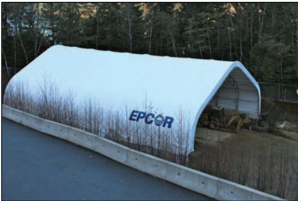
Sludge Storage Building at Britannia
