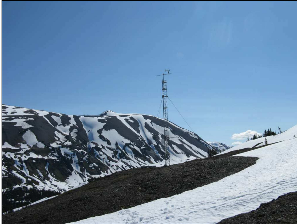
Plate 4-4. Unuk-Teigen 10 m Meteorological Station (June 2011).
