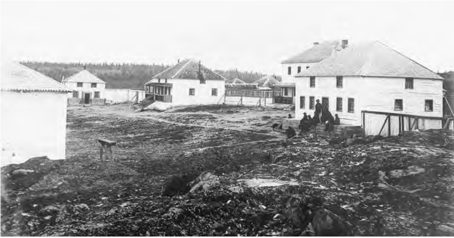
PHOTO 5.3 The Hudson's Bay Company continued to be the economic centre of Fort Chipewyan, despite heavy competition after 1870. | C.W. Mathers photo | Provincial Archives of Alberta, B.2952
