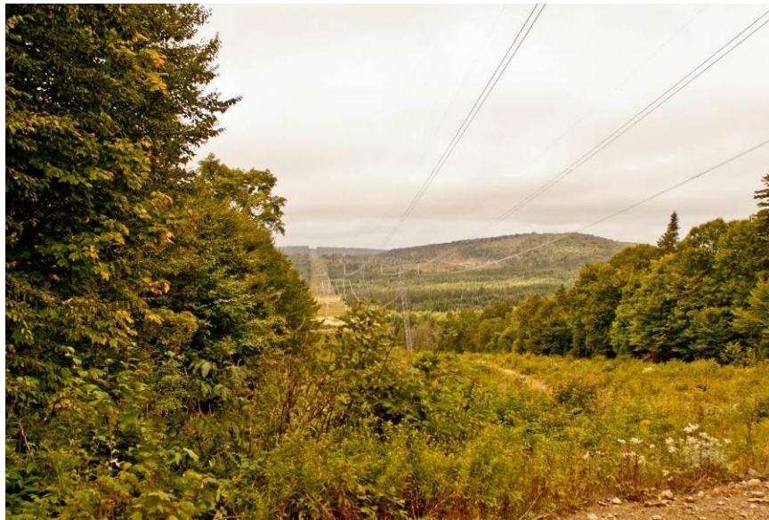
Figure 8.12.6 Photograph Taken Along Existing 345 kV Electrical Transmission Line, Looking Northwest Toward the PDA (Photo 3 in Figure 8.12.3)
