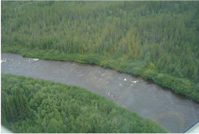
Photo 1. View of crossing at Site 48.
