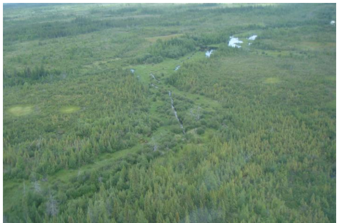
Photo 4. Downstream view of crossing at Site 46.
