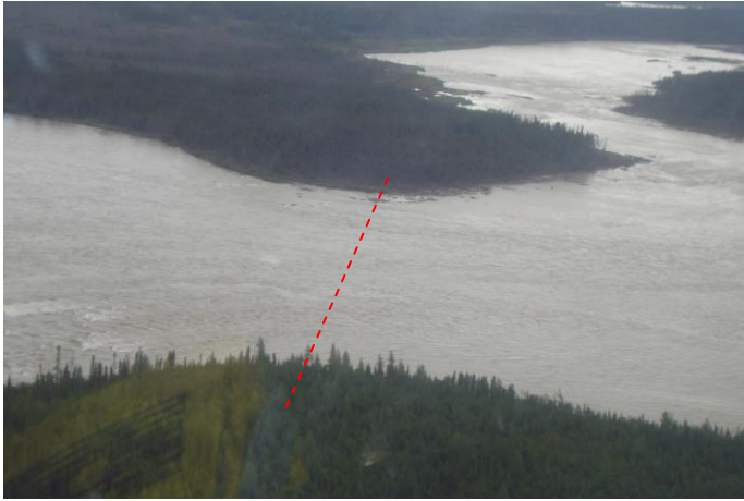
Photo 1. View of crossing at Site 1.
