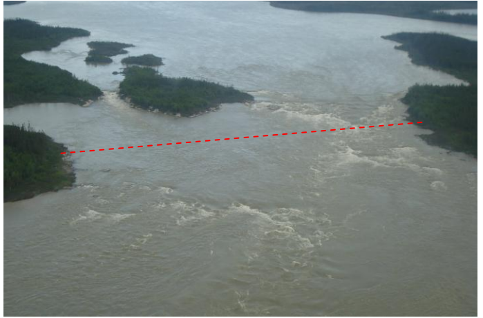
Photo 2. Upstream view of Site 2.
