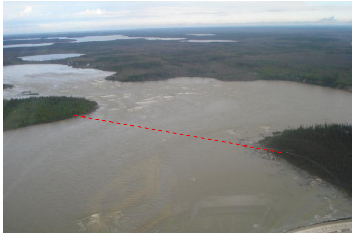
Photo 2. Upstream view of Site 1.
