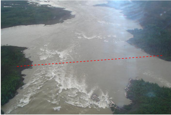
Photo 1. View of crossing at Site 2.
