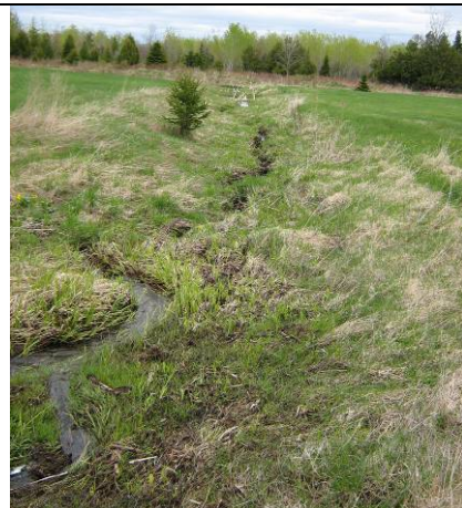
Photograph 10: New route of the north arm of the intermittent stream in the worksite area; looking northeast (May 2007).
