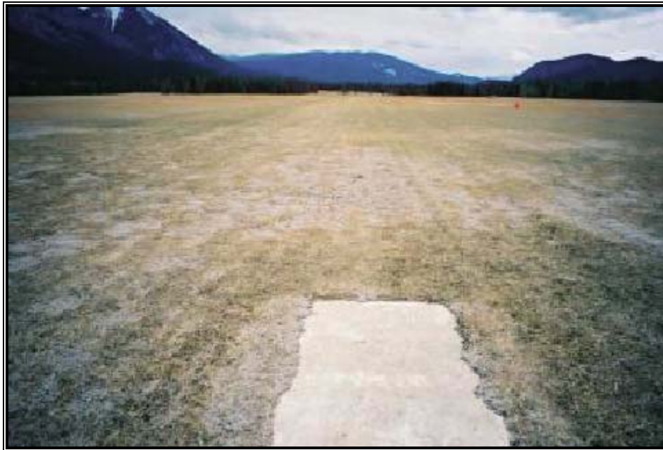
Photo 5. Concrete landing blocks at runway center –area of greatest landing impact
