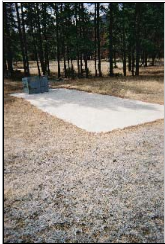
Photo 4. Concrete refuelling pad
