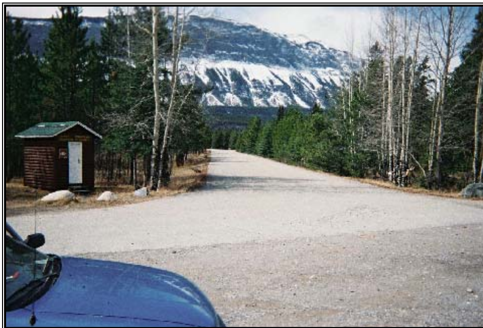
Photo 6. Paved access road and parking lot. Registration booth in the background.
