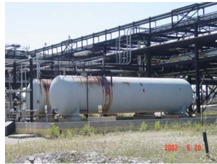
Photo 4 – Acid & Caustic Storage Area
