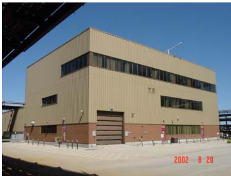
Photo 5 – Operations Building Common Services Clarifier Building & Plant D Filter Building
